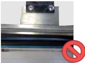
Gasket Too Tight
